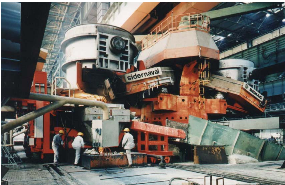
1996 WUHAN IRON & STEEL CO. (CHINA) CONTINUOUS CASTING PLANT
