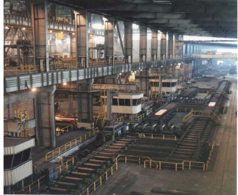
1985/ 1986 ALTOS HORNOS VIZCAYA (SPAIN) CONTINUOUS CASTING PLANT
